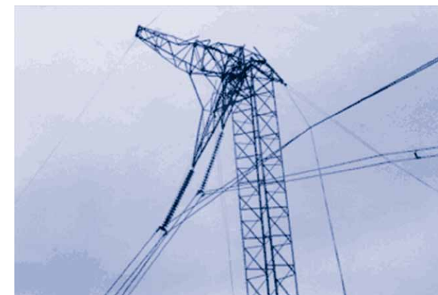
Field evidence of lattice tower failure at cross arms due to downburst event (Manitoba Hydro, 1999)
