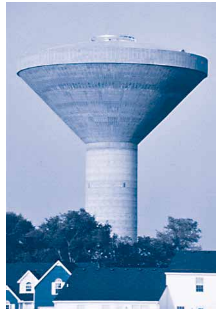
Example of a pure conical tank
